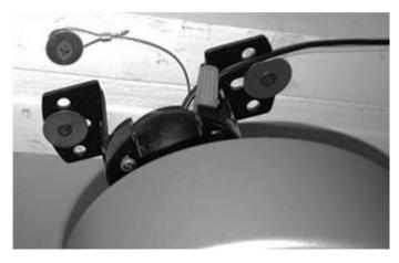
Photo 8: Safety cable attached near hanger
