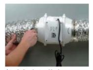
Attach the ducts with clamps.
