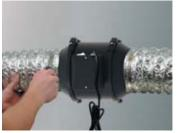
Attach the ducts with clamps.
