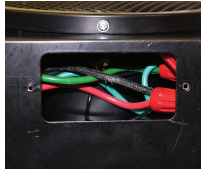
Figure 14: Wire connections carefully pushed into wiring compartment.
