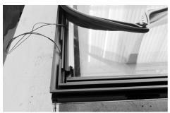
12. Pull the LED wires gently out of the bottom hinge pin.
