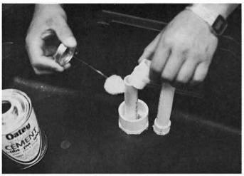
**Step 7**Use PVC pipe glue to glue the fitting to the <sup>3</sup>/<sub>4</sub>" fill line.
