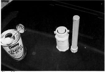
**Step 11** Screw the  $1^{1/2}$ " trap nut on the  $1^{1/2}$ " fitting and center the  $3^{1/4}$ " fitting carefully so you get a good watertight seal. Now is a good time to flush your new system by turning on the water for awhile to flush line.
