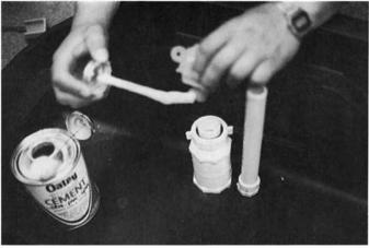
**Step 12**Using pipe thread sealer or teflon tape treat the threads on the valve. Teflon tape is preferred.
