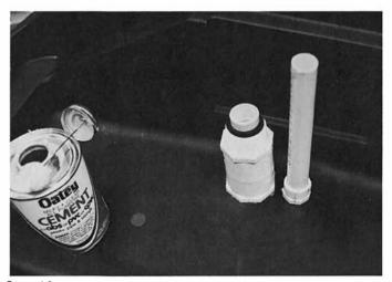
**Step 10** Put the rubber washer back on the  $^{3}/_{4}$ " female fitting. Slide on and into the groove. Make sure it is lying flat on top of the  $1^{1}/_{2}$ " fitting so you get a good seal.
