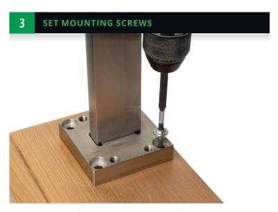
Images in steps 2-3 show GRK RSS 5/16 x 5-1/8", an alternative screw to the Cable Bullet post mounting screws (1/4" SS star drive socket head cap screws).
