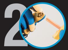
Check the refrigerant line end & ensure it is properly cut & cleaned. Put the flare nut on the refrigerant line & hold the line firmly.
