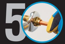
Thread the flare nut onto the male fitting and tighten using correct tools to equipment manufacturer torque specifications.
