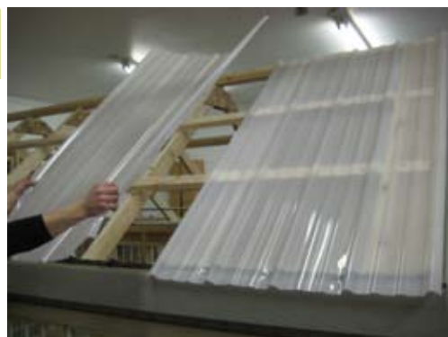
Continue with roof.
