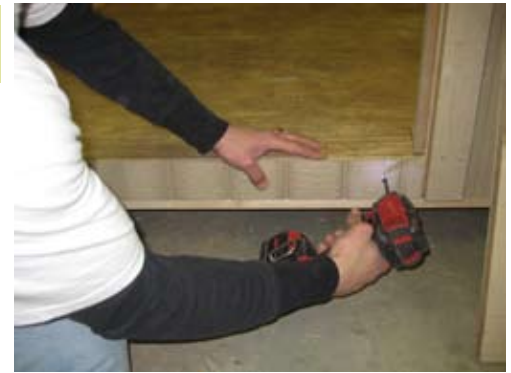
Next install 3" siding strip below door opening and secure with 1 1/4" screws.
