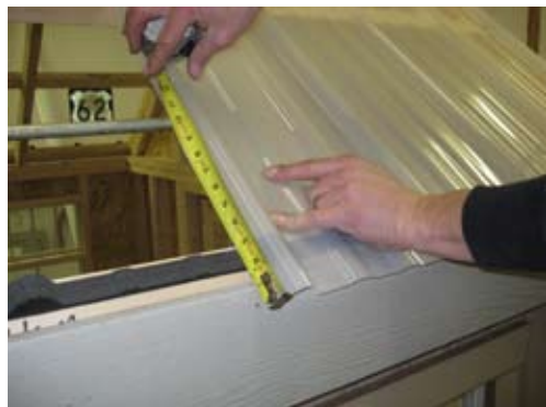
Continue with roof. 1" overhang
