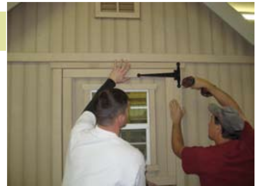
Next install top door first and make sure you have a 1/4" space on top as shown. Secure with 2 1/2" Black Headed Screws.
