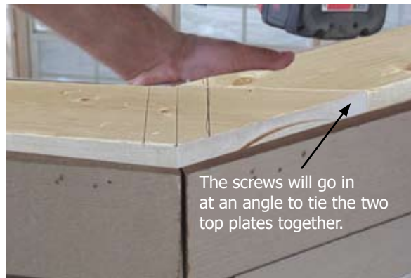
19. Make sure the inside corner is in place and secure with 2 1/2" Zinc screws as shown.
