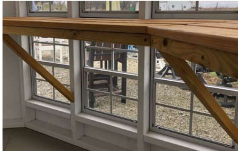
38. The short braces will be installed on end shelves.
