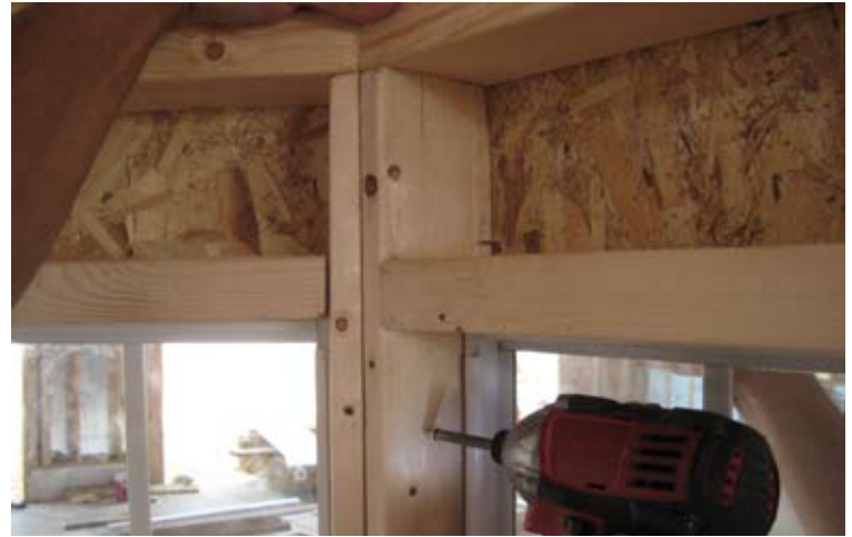
19. Make sure the inside corner is in place and secure with 2 1/2" Zinc screws as shown.
