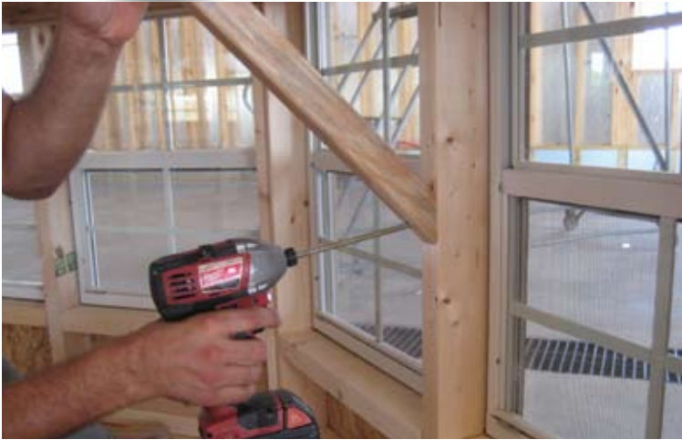
37. Next install brace as shown.
