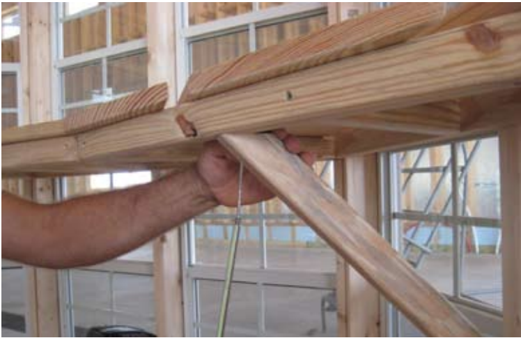
39. If wood wants to split use 1/8" drill bit and drill hole where screw is shown to go through.
