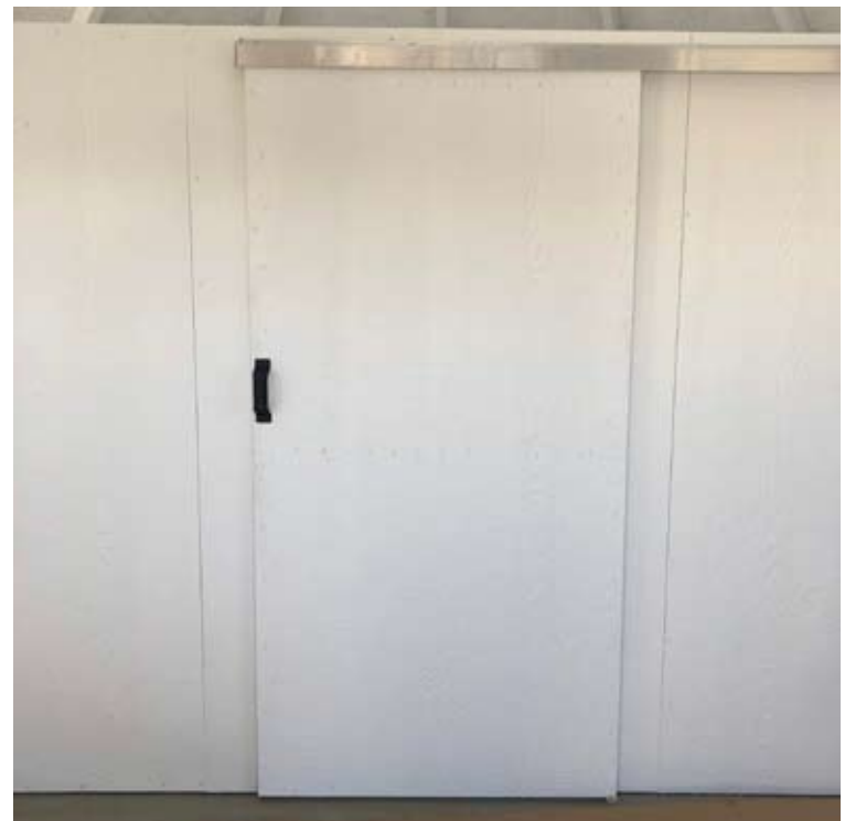
30. Attach the trolley wheels to the top of the door. Also attach the door handle to the door. Hang the door on the track.
