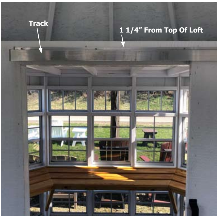
29. Then locate the track hardware for the sliding door. Attach the track to the header that is above the door opening, 1 1/4" from the top of the loft.
