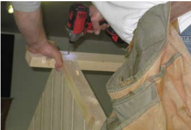
63. Install last row of purlins.
