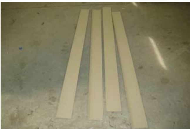
71. Next locate the 7/16 siding for soffit.
