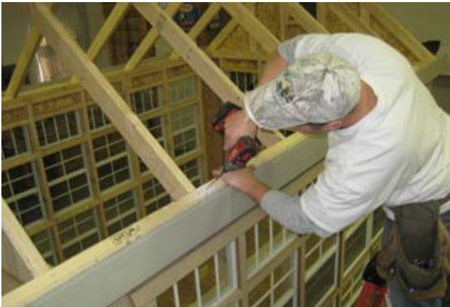
57. Secure with 2 1/2" screws.
