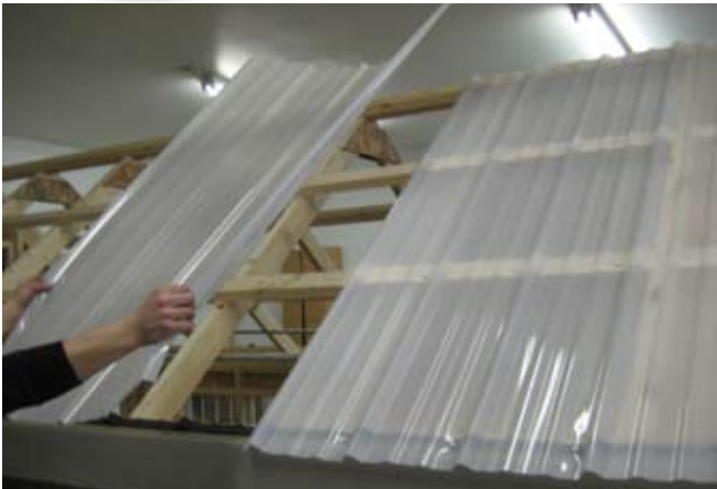
134. Continue with roof.
