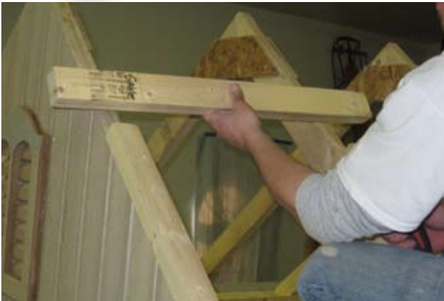
61. Continue with purlins.
