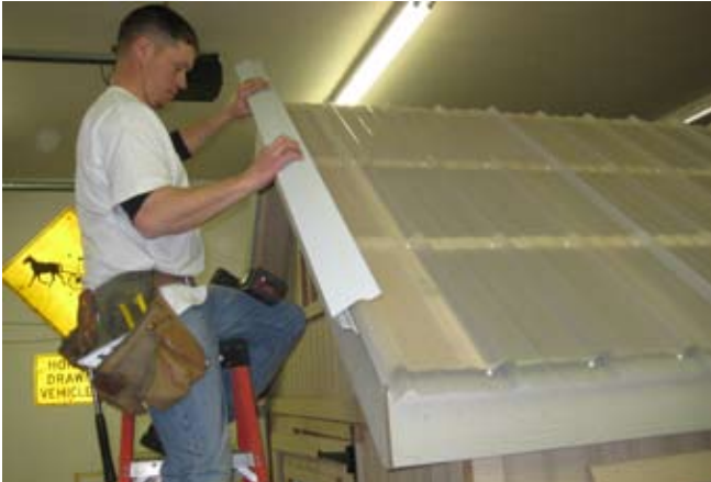
140. Install rake cover with wider side on top.
