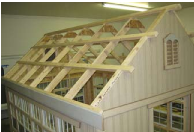
65. Purlins are completed.
