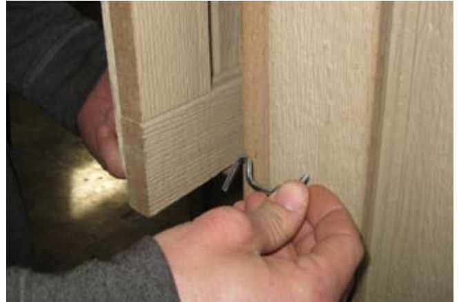
105. Open top door to locate where to install hook and eye.
