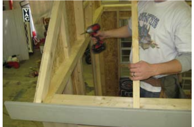
50. Next set trusses.
