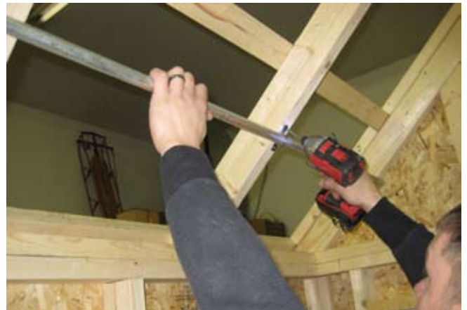
125. Use 1 1/4" screws to secure pipe in place.
