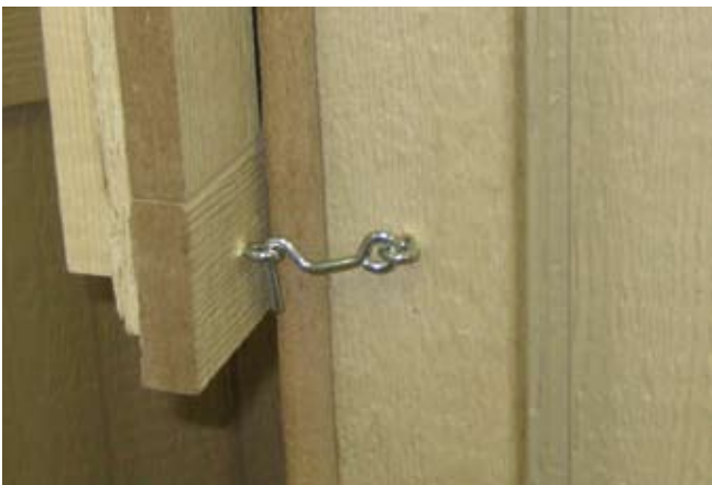
108. This is what it should look like when completed.
