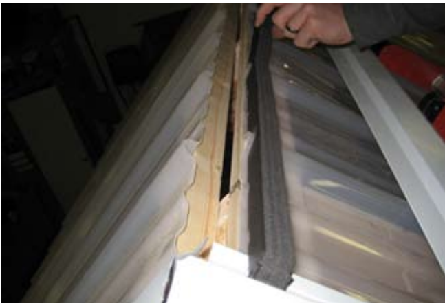
148. Next install ridge enclosures 2 1/2" from peak.
