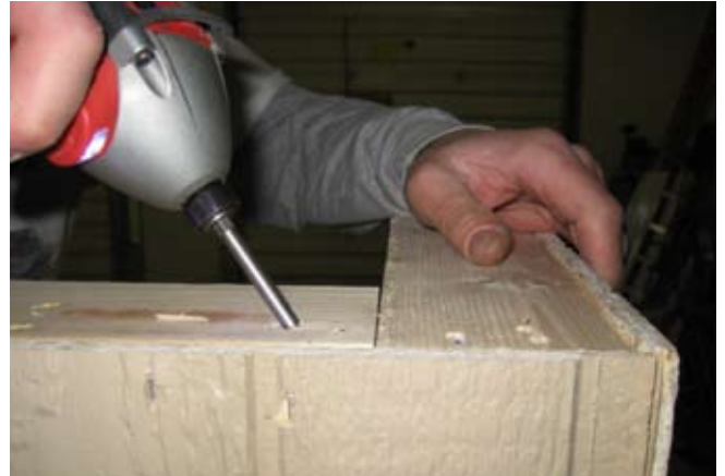
26. Secure with 2 1/2" Screws on an angle.
