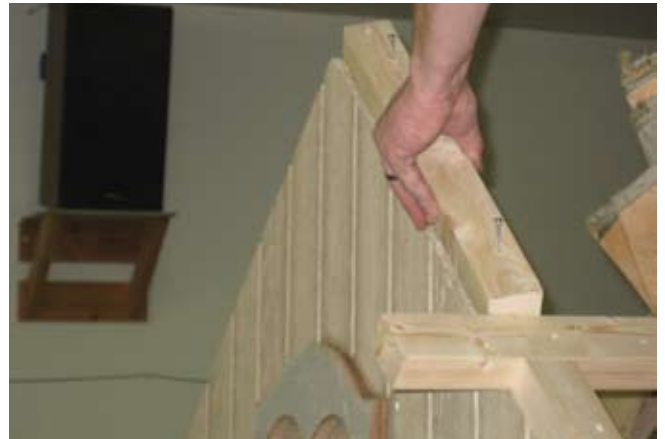
62. Install last bird block as shown.
