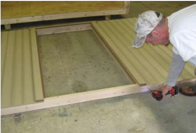
27. Remove 2x4 plate underneath door.
