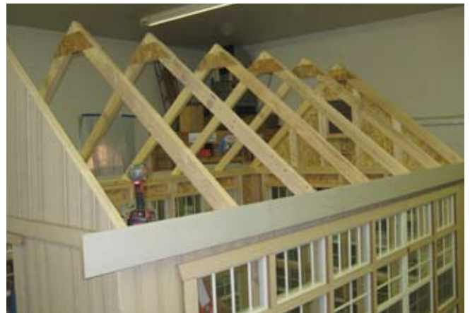
52. Trusses are completed.
