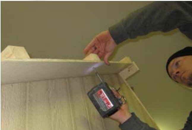
73. Secure with 1 1/4" screws.
