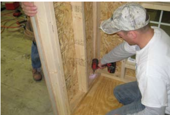
29. Apply pressure on outside and secure with 2 1/2" screw.
