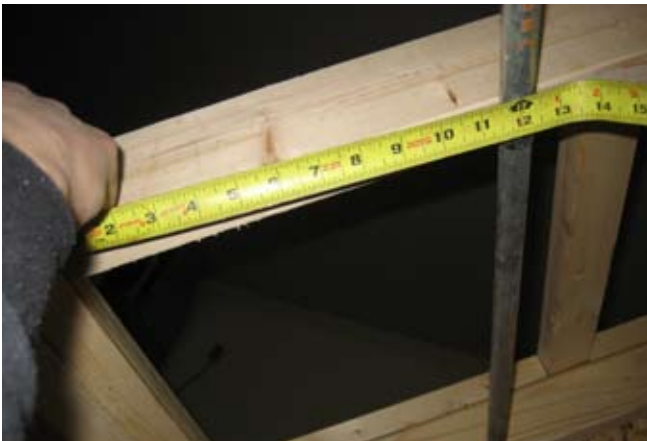
124. Measure 12" from top plate to where pipe should be fastened.
