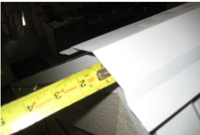
150. Next install ridge cap, over hang cap 1".
