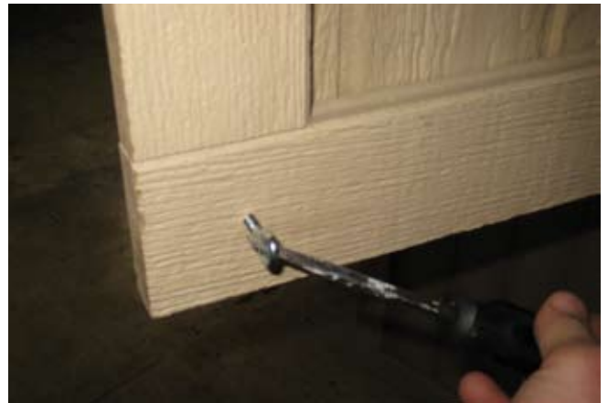
107. Install eye where hole was drilled.
