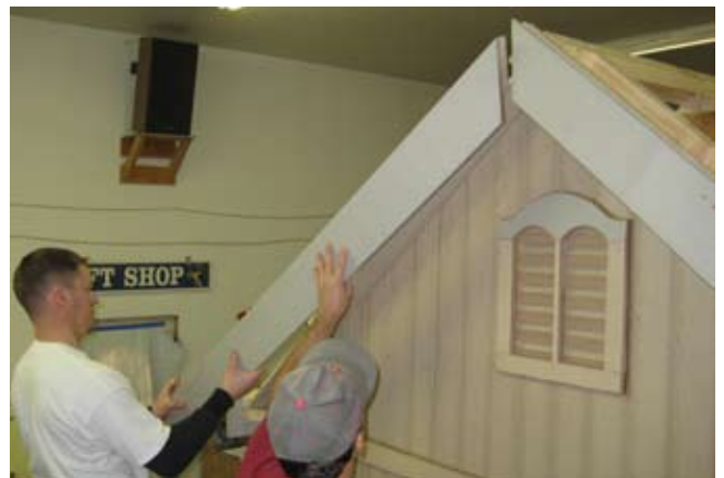
78. Install rake on left side and repeat from first one.
