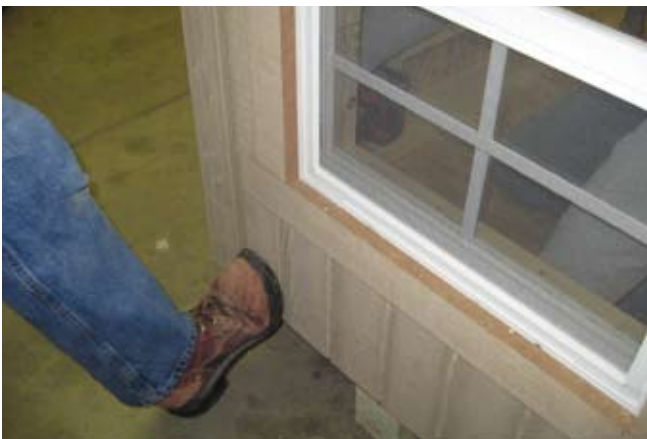
23. Apply pressure on outside while fastening with 2 1/2" screw from inside as shown.
