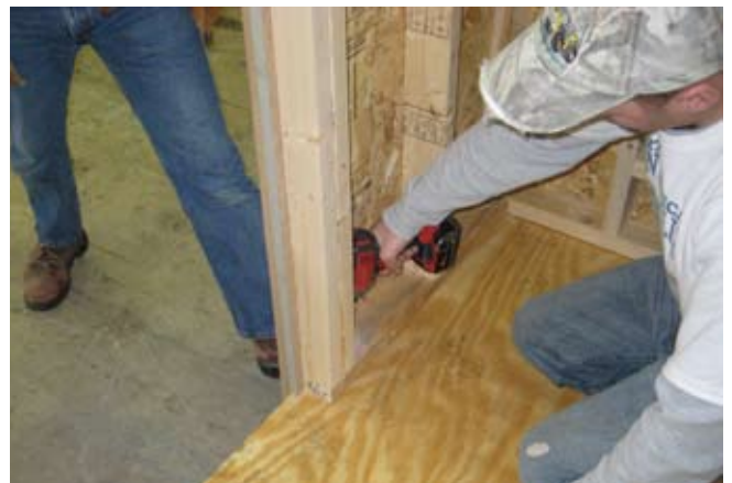
30. Secure corner with 2 1/2" screw.
