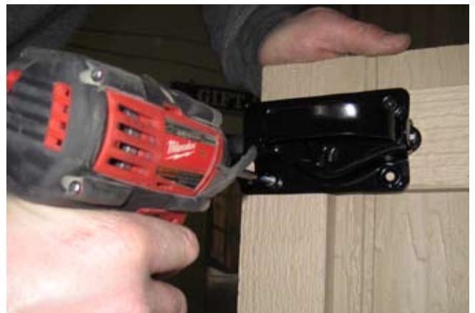
96. Secure with 1 1/4" black headed screws.
