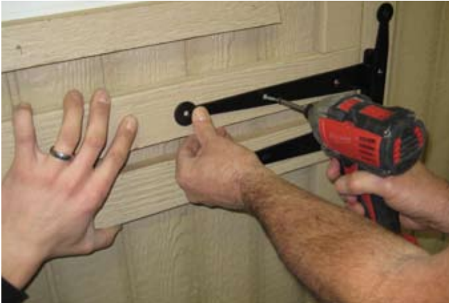
91. Secure with 2 1/2" black headed screws.
