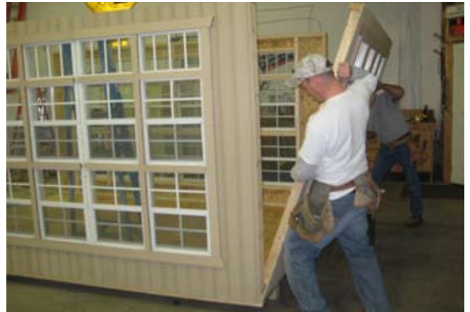
22. Next install end wall.
