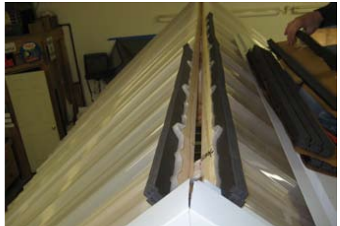
149. Continue installing enclosures.
