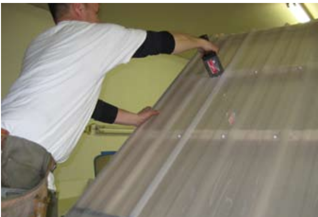
138. Continue with roof as shown.
