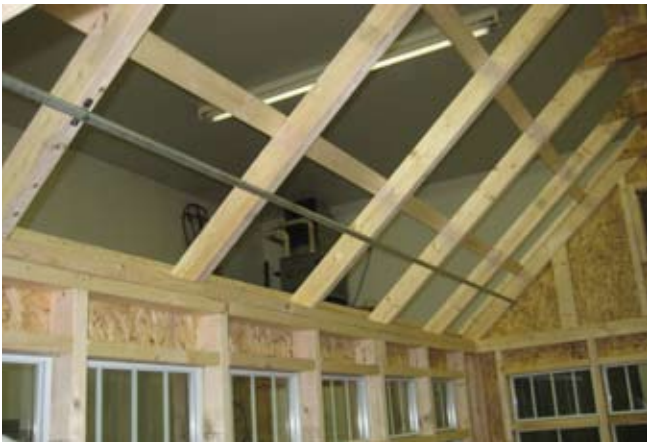
126. Install C-clamp on every truss.
