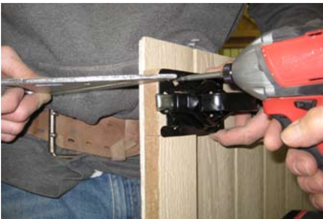
95. Make sure you use angle square as shown, so latch is flush with trim.
