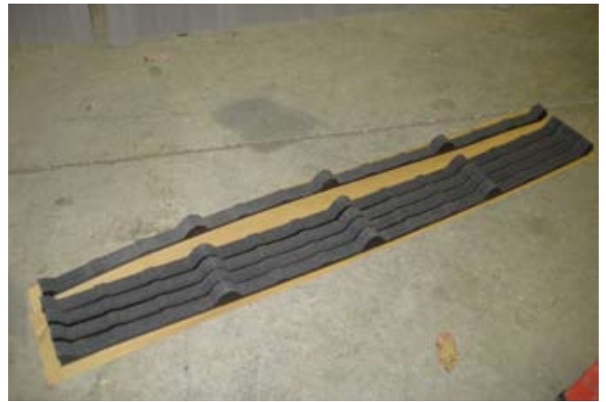
127. Next locate upside down rubber closures.
