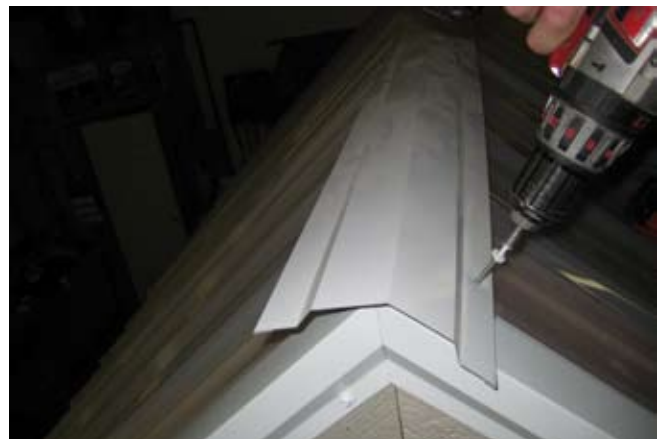
151. Secure ridge cap with 2" white screw beside every rib.
