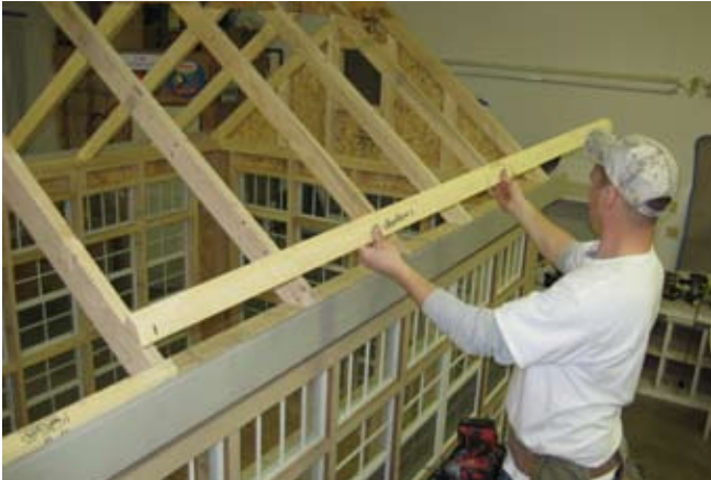
55. Continue with purlins.
