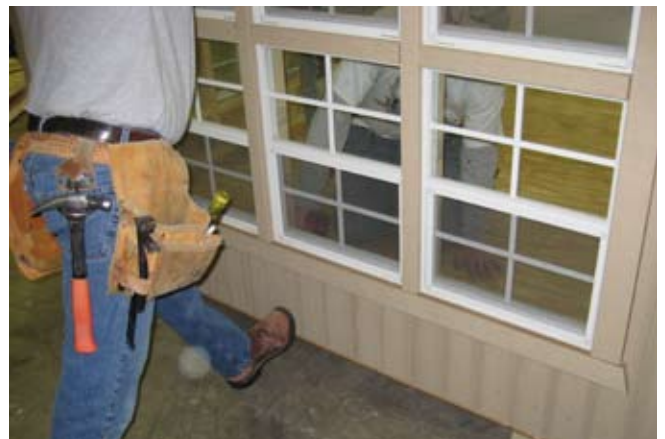
24. Apply pressure on all walls as shown before securing with 2 1/2" screws.
