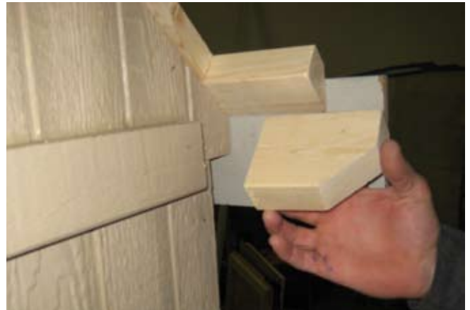
68. Install rake blocks as shown.
