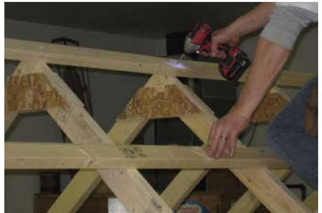
64. Secure with 2 1/2" screws.
