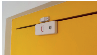
Magnet positioned flush with main sensor
