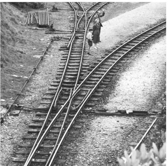
VoR pointwork at Devil's Bridge, circa 1960. The tongue rails slide on special baseplates, firmly fixed with 'tirefond' bolts.
