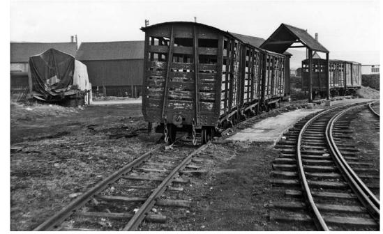
Although there is a clear contrast of maintenance standards between the siding and main line on the 2ft 6in. gauge track in Welshpool yard on 26 March, 1956, both are clearly 'Fit for the purpose'.
