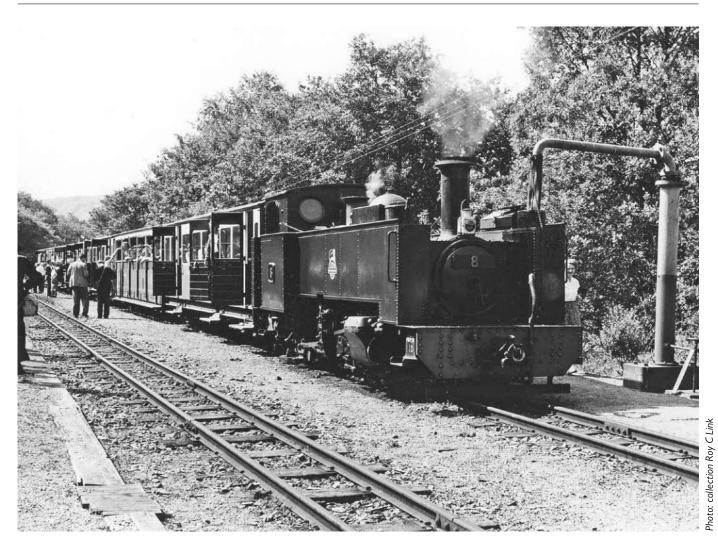
Classic early 1950s Vale of Rheidol. An up train, hauled by No.8 (later, in 1956, named Llywelyn) takes on water at Aberffrwd. The spiked flatbottom rail, with steel baseplates on timber sleepers, is clearly visible in the foreground. Joints are staggered – note that the heads of the fishplate bolts face inwards.
