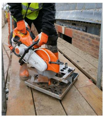
Using the Large Jig in this way means that the bricklayer or labourer is safely away from the running cut-off saw and the risk of flying bricks. With the bricks sitting up off the floor, the cut is well away from the feet, legs and body of the operator and there is less strain on their back.
