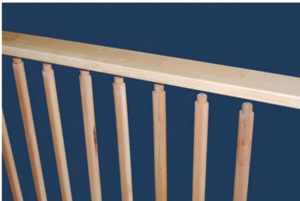
3. Fit the second rail. Engage the first rung on either end and progressively fit each rung until all are seated.
