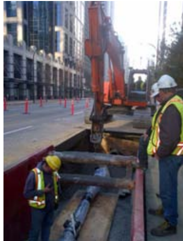
Figure 6: Sliplining on Georgia Street
