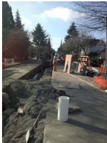
Figure 5: East Pender Street Transmission Main Construction
