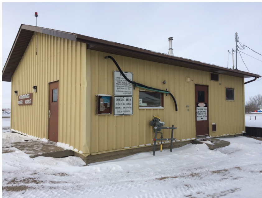
Strasbourg Water Treatment Plant Building and Truck Fill Station
