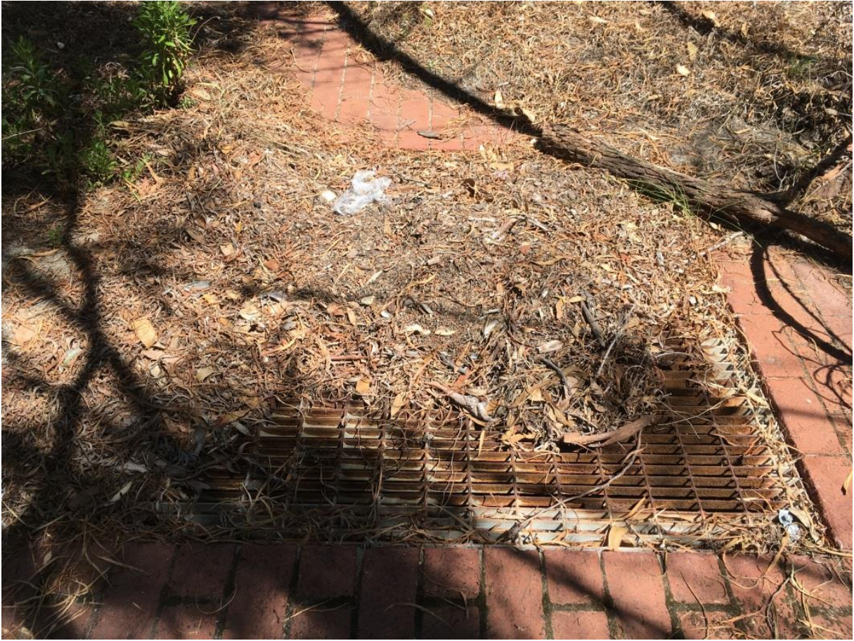
Figure 11-2: grate in Trevor Gribble Park compensation basin with leaf litter and sediment sitting on top.
