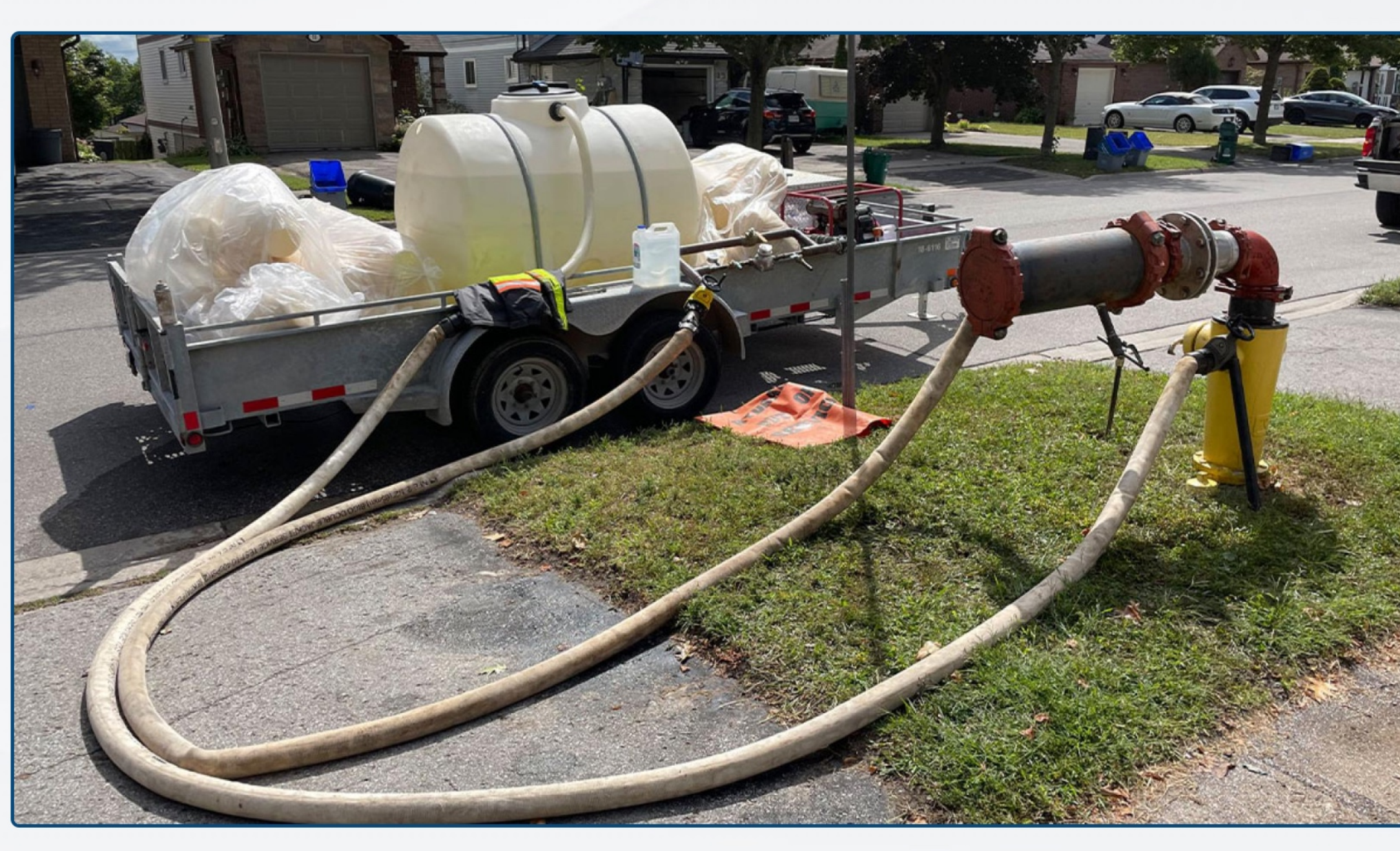
Equipment used to launch swabs into watermain.
