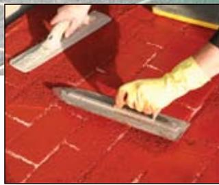
2. Colour Hardener is then applied to the surface of the concrete and trowelled in.
