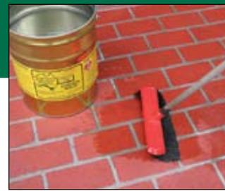
4. Finally, a sealer is applied to protect the surface from staining and to give you an attractive and durable finish.
