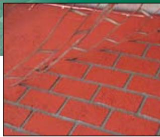
3. After the concrete has been left to dry sufficiently, the paper stencil is removed to reveal the required pattern.
