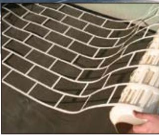
1. The concrete is poured to a minimum thickness of 100mm. A paper stencil is then laid on top of the concrete.
