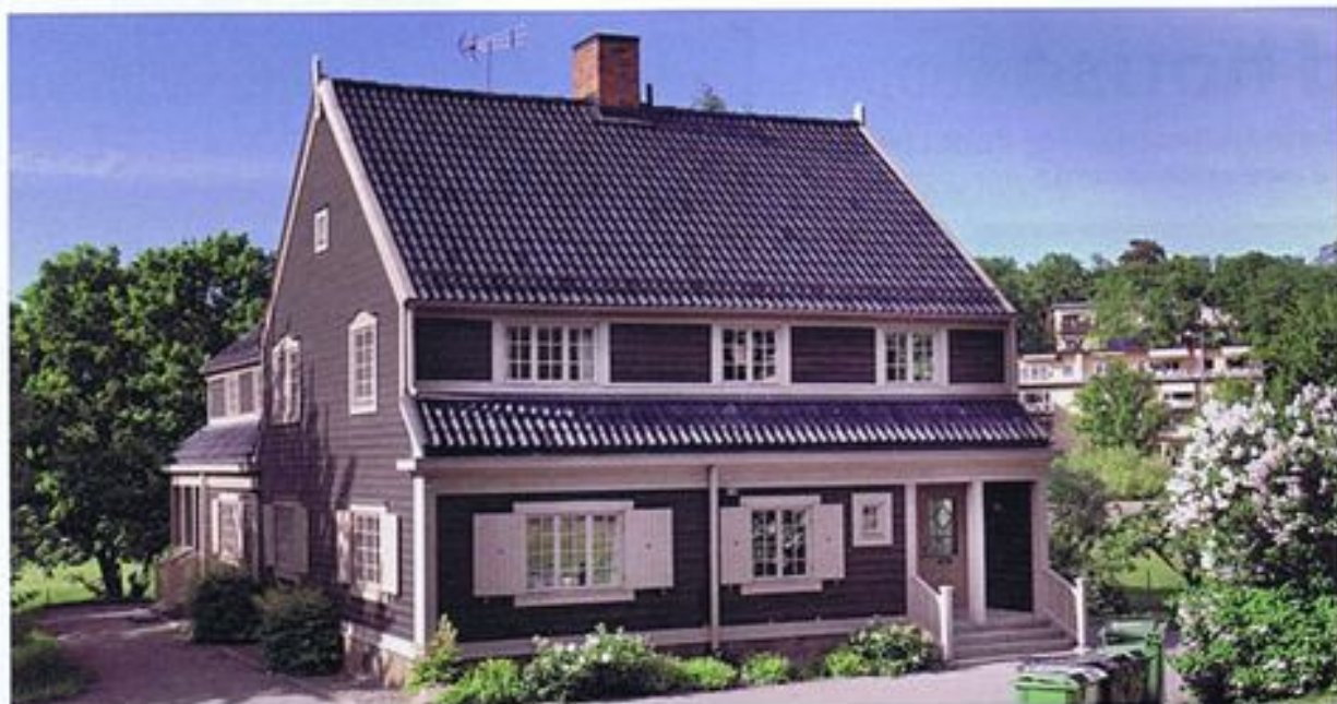
Hallarbergs Country House: pine timber houses can last many centuries when painted with linseed paints.
