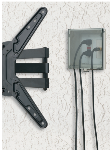
TV bracket mounts near box (allow for access to cover)
