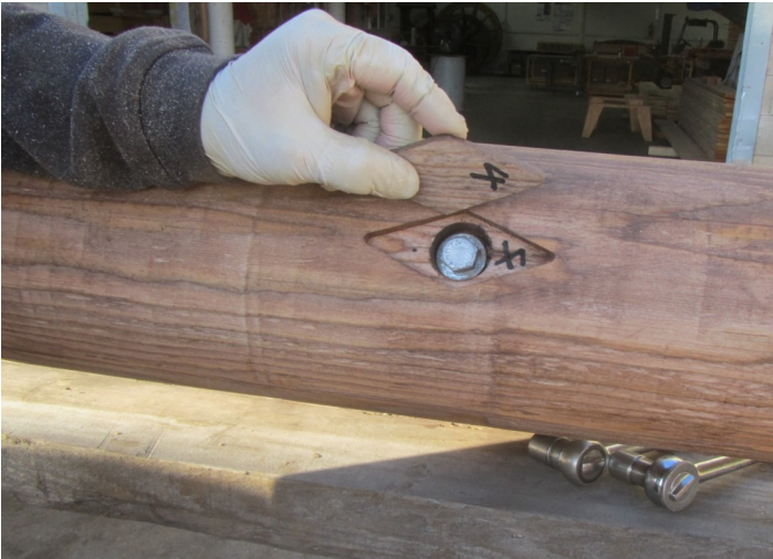
19. Fasten wood pegs to cover the holes with nails. Match the number or alphabet.
