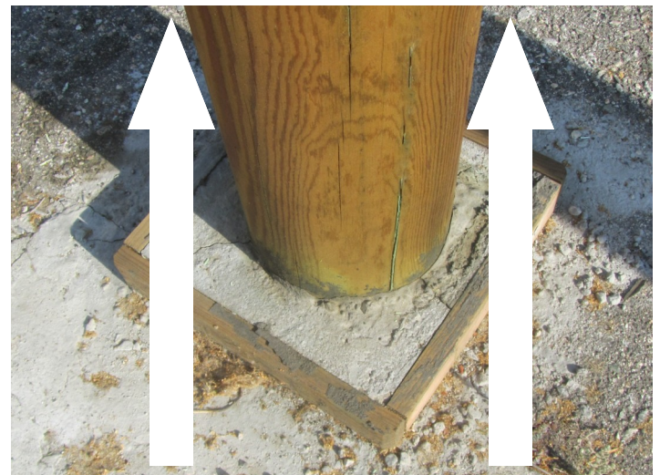
10. Insert square frames and tie them to the NUKI. Skip this step if you prefer not to use them.
