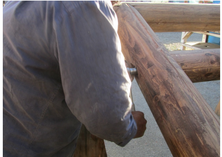
20. Fasten the loose lag bolts from sides (steps 7 and 8).
