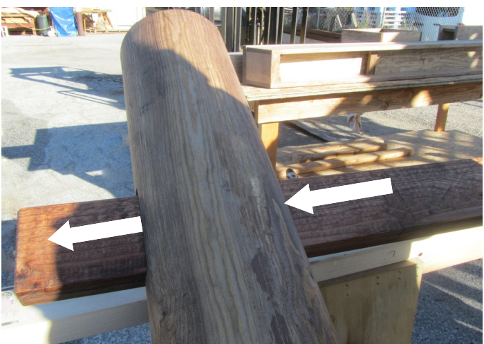
5. Insert a NUKI through pole holes. Do it one pole (HASHIRA) at a time.
