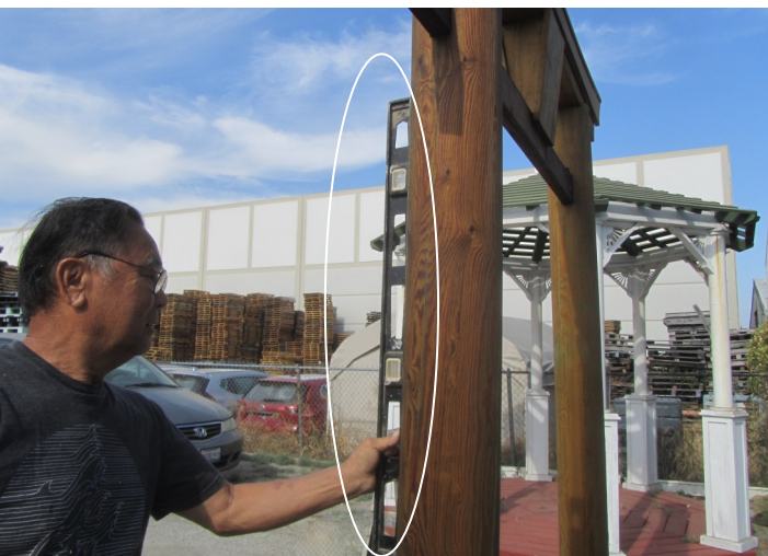
19. Check the level from front or back. Adjust the pole positions if not level.
