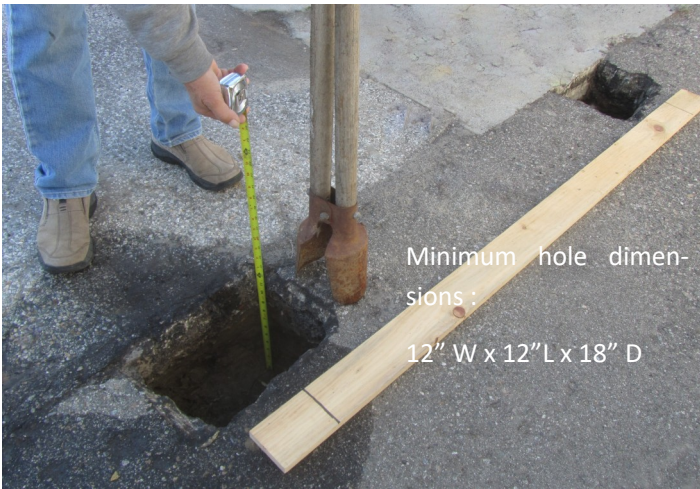
1. Making two holes for Torii poles. Remember that you need to set minimum 6" with cement.(See marks on posts.)
