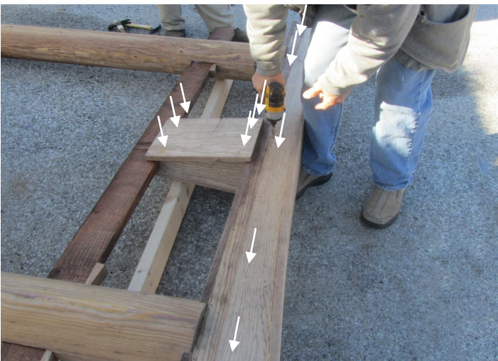
17. Fasten the Top KASAGI and Bottom KASAGI with small screws. Fasten the GAKUZUKA and the NUKI.
