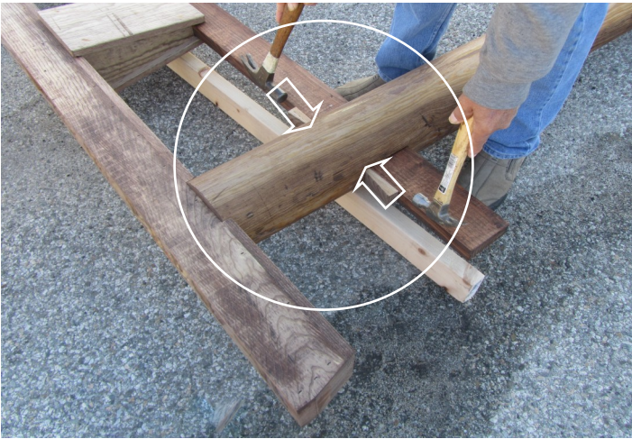
15. Gently hammer both KUSABI at the same time until a part of the KUSABI fills the hole; it will permanently lock the NUKI in place. Do the same for the other side of the NUKI.
