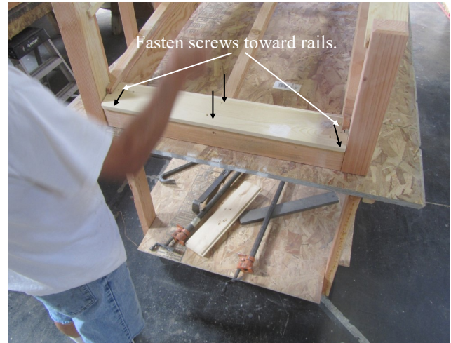
12. Turn it over (see 11) and fasten it with small screws.
