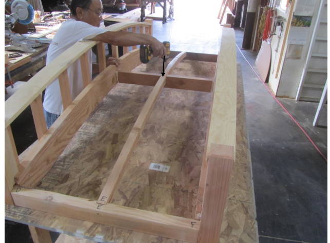
8. Fasten the floor joists with a large screw.
