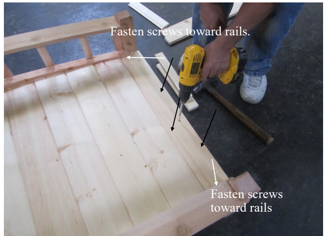
16. Fasten the end floor board with small screws .
