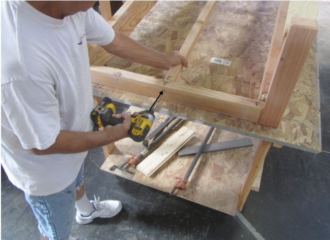
7. Fasten the end frame and the large floor joist with a large screw. Do the same for the other end.
