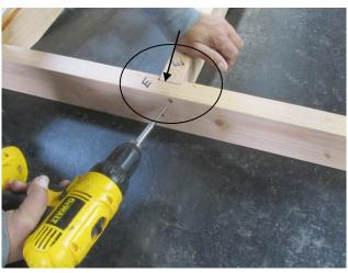
7. Fasten the end frame and the large floor joist with a large screw. Do the same on the other end.
