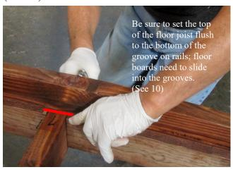
5. Fasten the small floor joist with a small lag bolt. Do both end.
