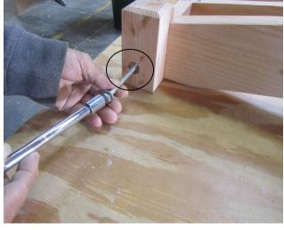
2. Fasten the rail and end frame with a large lag bolt.
