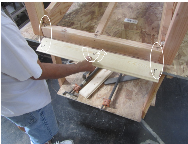
11. Find an end floor board with matching number.
