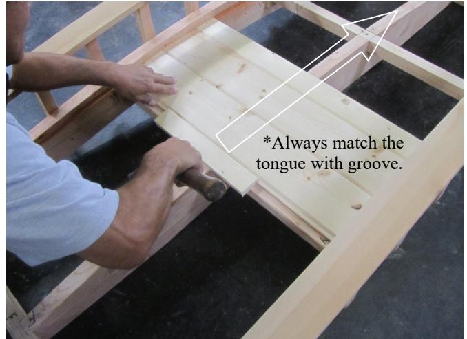
14. Continue to slide in more floor boards.
