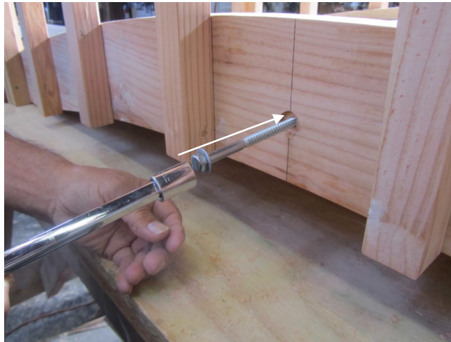
9. Fasten the small floor joist and rail with a small lag bolt .
