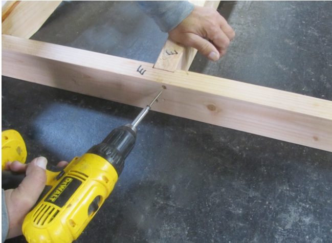
7. Fasten the end frame and the large floor joist with a large screw.
