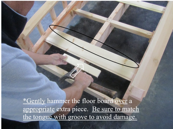
13. Check the tongue and groove of the end floor board on the other end and slide in floor boards one at a time. The tongue of the floor boards should go into the groove.
