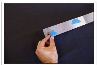
Tape the Rivnuts onto the Backing Plate.
