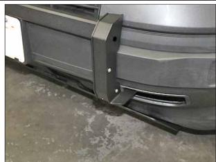
Attach the light bar assembly to the Chassis Mounting Brackets by inserting (1) 1/4"-20 x3/4" Button Head Bolt into each of the open holes shown above. Remember to use a drop of blue Loctite on each bolt before fastening. Leave the Top Hole open for the next steps. Repeat on the opposite side.
