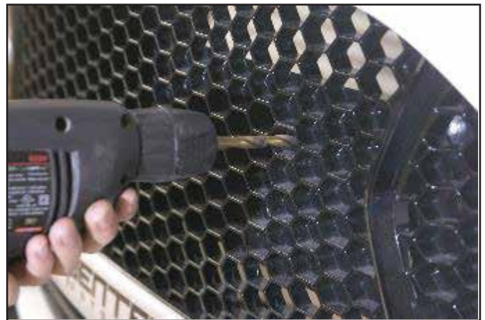
Drill through grill with 3/8" Drill Bit.
