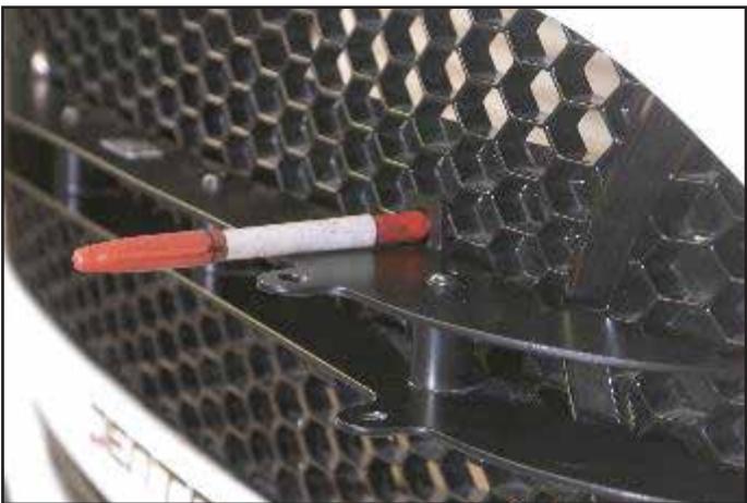
Mark center of hexes for drilling.
