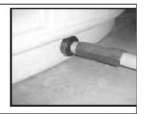
The spa drain valve assembly consists of a garden hose connector with a twist on/off valve and a safety drain cap. It is located behind the waterfall (outside) at the bottom of the spa.
