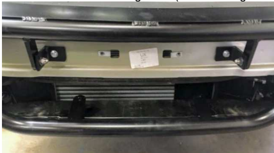
Figure 16: Temporarily Install to Verify Alignment of Lower Attachment
