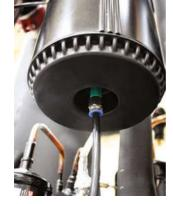
Liquid water droplets coming from the line to the inlet of the dryer are separated by the inlet filter and drained. Filter auto drains have manual valves on them. This allows the system to be depressurized when these filters go to service.
