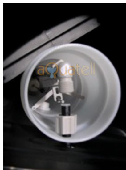
To attach the brine line to the brine tank you will first insert the tube insert into one end of the brine line. Be sure to push it all the way in. Then pass this end of the brine line through the upper hole in the brine tank and through into the brine well. Slide the hex nut onto the brine line and then insert the brine line fully into the threaded elbow of the brine float. Now tighten down the hex nut until it is snug making sure that the brine line is held firmly in place.
