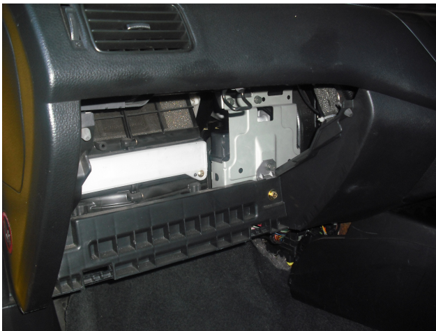
Figure 3 – Factory ECU Location (Glove Compartment Removed)
