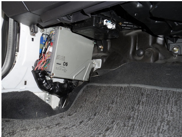
Figure 1 – Left hand side kick panel showing ECU Location
