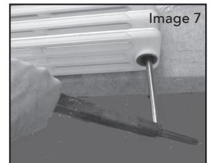
12. Once the joins are satisfactorily tightened you can fit the blanking plugs, bushes and gaskets. Please note these items are also left and right handed to avoid cross threading.
