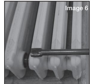
10. The two nipples should now be tightened alternatively to keep the radiators parallel. The key should be kept in a central position in the waterway whilst turning. Tighten the first nipple with 2 turns only, pulling the two sections together. Repeat the process alternating between nipples, until both sections are joined hand tight.
