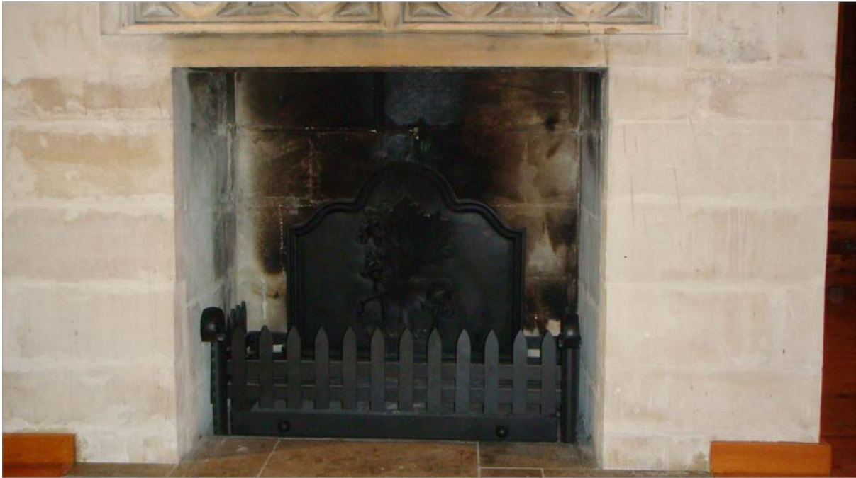
The fireplace with 1000X500mm Basket and Back Plate
