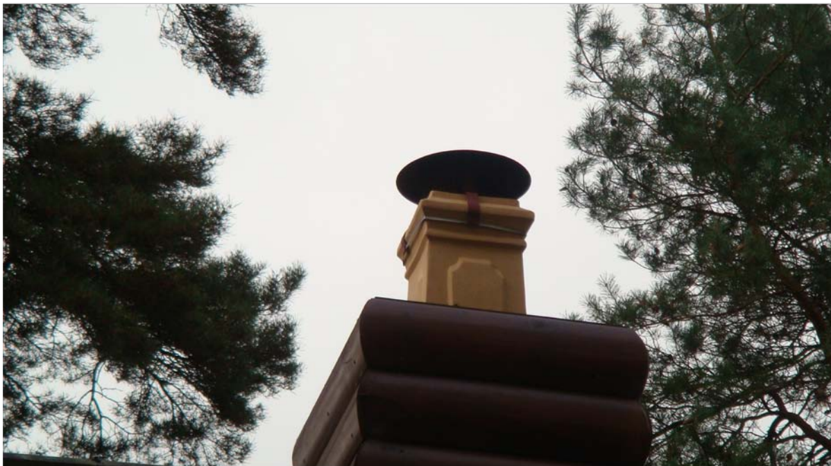
Chimney Sack terminated with tapered square pot 206-180mm and 206mm rain-hat cowl
