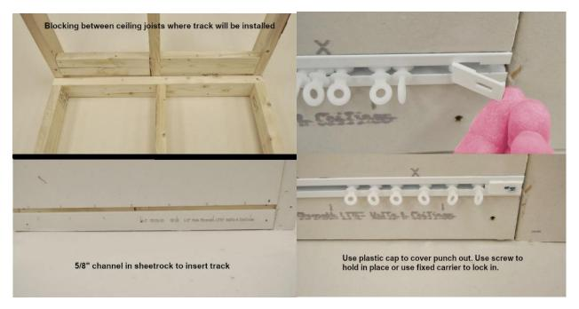
Screw the track approximately every 24". If a screw is needed where a hole is not pre-drilled, use the center indentation line on the track as a guide to drill a small pilot hole. Use trim head screws and take care not to score the channel. The flanges on the track will cover the edges of the sheetrock with no compound (mud) needed.
