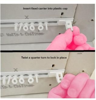
The square punched area on one end will allow slides to be added or removed. Cover with the plastic cap. Either screw the cap in place or use the fixed carrier to lock it in place.
