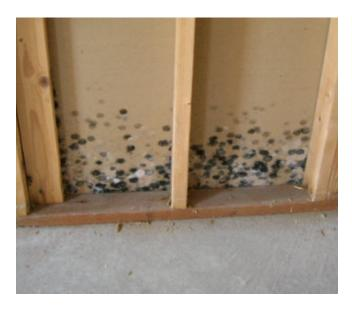
In the above picture the mold was not visible until the drywall was removed from the wall. In a new home the concrete will release moisture for 1.5 to 2 years. This picture illustrates how the wood has absorbed the moisture from the concrete and drawn it up into the space. With this additional moisture and no air movement, the mold thrives.
