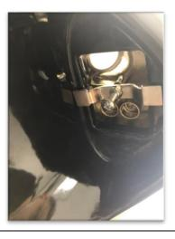
11) Feed the A203 Shower Hose and Head through the hole on the Vacuum Breaker plate and cap on the plate as well.
