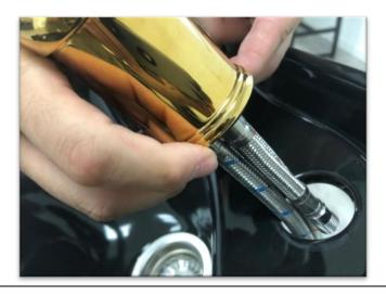
8) Replace the metal collar and matching rubber gasket onto the faucet; tighten back on the brass fitting.
