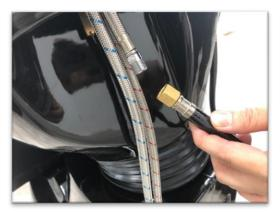
13) Feed the lines of the faucet into the hole of the base.
