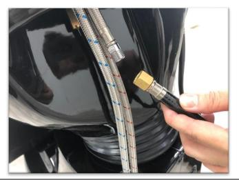
15) Feed the lines of the faucet into the hole of the base.
