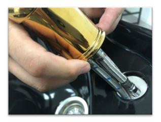
10) Replace the metal collar and matching rubber gasket onto the faucet; tighten back on the brass fitting.
