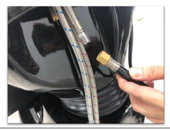
15) Feed the lines of the faucet into the hole of the base.
