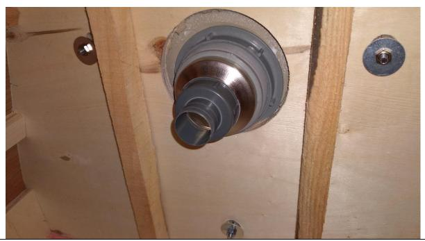
10) Take the Drain Hose and attach that to the bottom of the Drain. Please note that the Grey Drain Adapter in the previous pictures in steps 7 and 9 is used for a different type of drain hose and is determined by you and your plumber.
