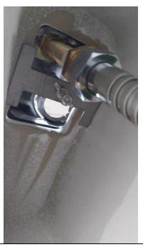
12) Take the flexible hose from the Vacuum Breaker Assembly and feed it upward through the round hole of the Vacuum Breaker Plate and attach the Sliver Shower Head.
