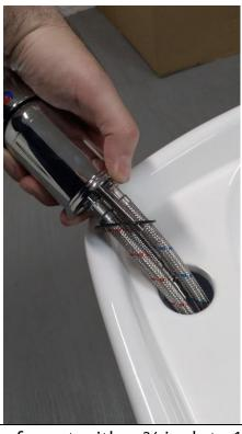
14) Connect the Silver Shower Head and Hose to the faucet with a  $\frac{3}{4}$  inch to  $\frac{1}{2}$  inch (female to male) NPT brass adapter fitting.
