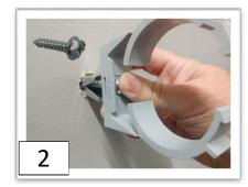
Insert Wood Screw through Clamp and Tighten. Insert Toggle into Hole for Drywall Installation.
