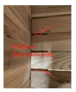
Install the bench leg supports on each side and secure with 2x '4\*40mm Screws'.
