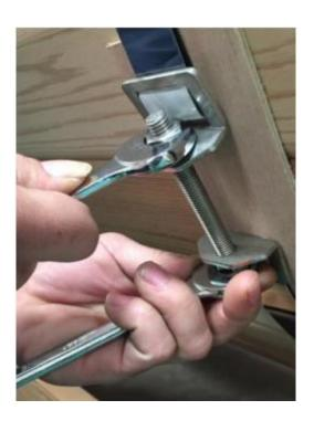
12.Install the benches inside in the barrel. Place the long benches onto the sides of the barrel using the supports at the front and back panels. In the center on the bench underneath, install the 20cm 'Inside bench support beam' onto the side of the barrel wall using 2x '4\*40mm Screws'. Then screw the bench from the topside down into the support beams.
