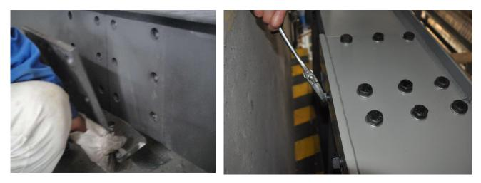
5.3.3.3 After installing the connection plate, two sets a half weighing platform consists of a large weighing platform, which finish the assembling of weighing platform
