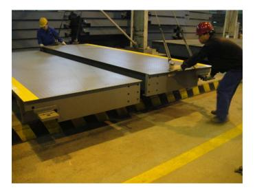
Note: Please find out the 2pcs same serial No. weighing platform out and find out the same serial No. connection plate out. Then install them together. Different serial No. weighing platform can't be installed together.
