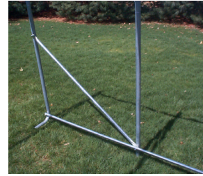
Structural wind brace on each corner
