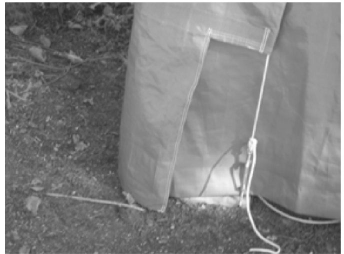
Turnbuckle on Main Cover goes on the Outside of the End Panel/Zipper Door
